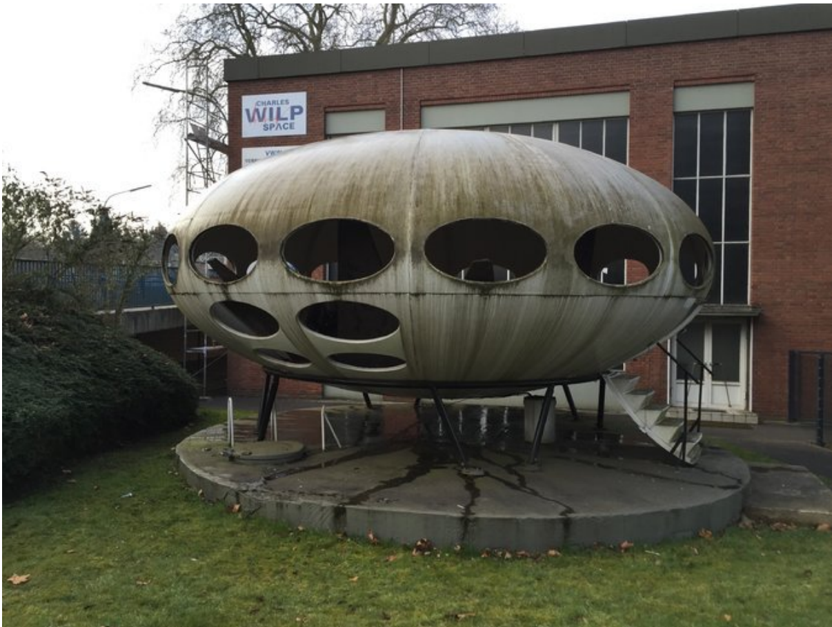
A 1960s Futuro, a white fiberglass pod made in Germany and meant to serve as a portable ski lodge, suffered damage while stationed outdoors for decades at various sites in Germany.
